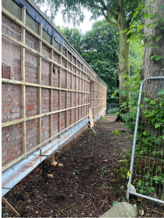
Hempcrete Installation - preparation
