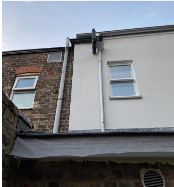
External Wall Insulation
