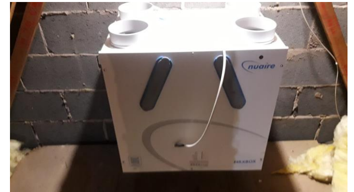
Mechanical Ventilation Heat Recovery (MVHR)
