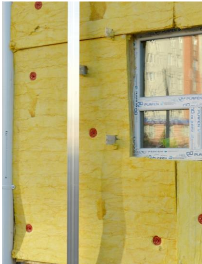
External Wall Insulation
