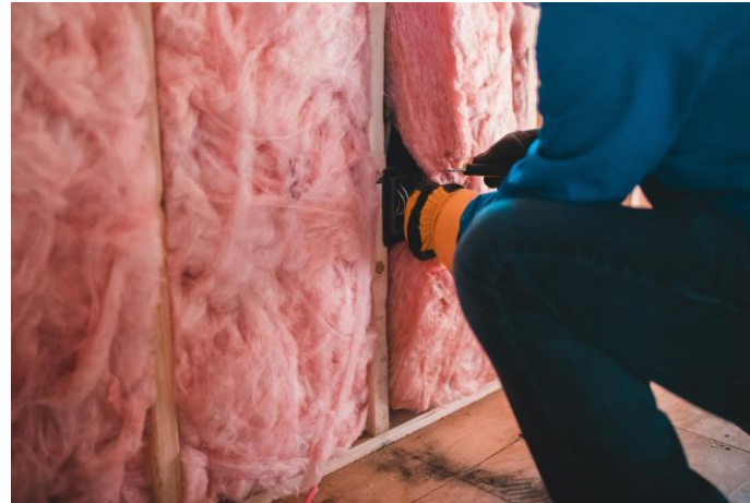
Internal Wall Insulation
